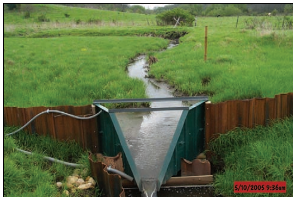
Figure 33: Down stream site (H2) with sheet piling wing walls
