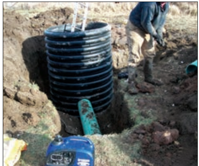
Figure 18. A 5-foot-diameter culvert was installed to allow access to in-field subsurface tiles.
