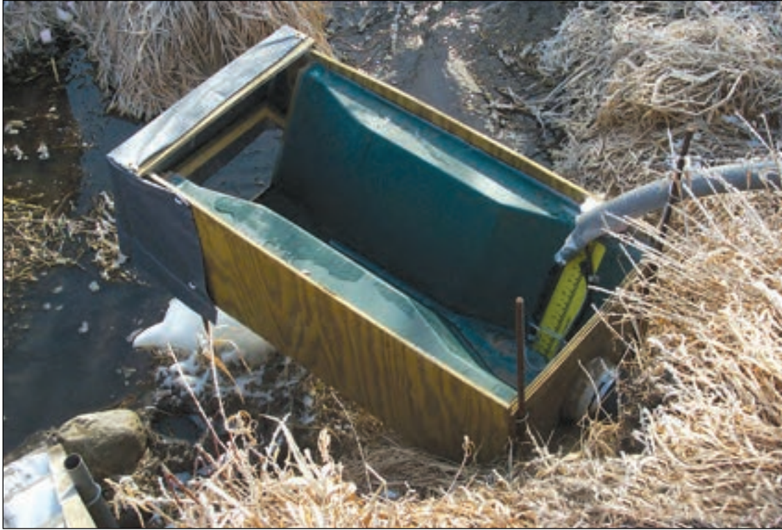
Figure 20. Extra-large, 60-degree, v-throat, trapezoidal flumes were used to compute discharge at the outlets of subsurface tiles. The insulated plywood cover was removed for this photo.
