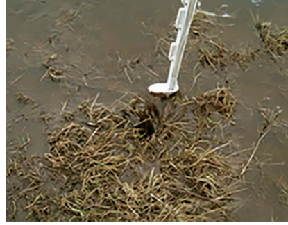
Figure 10. Water entering blowout
