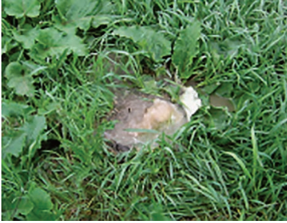
Figure 9. Water gushing from blowout
