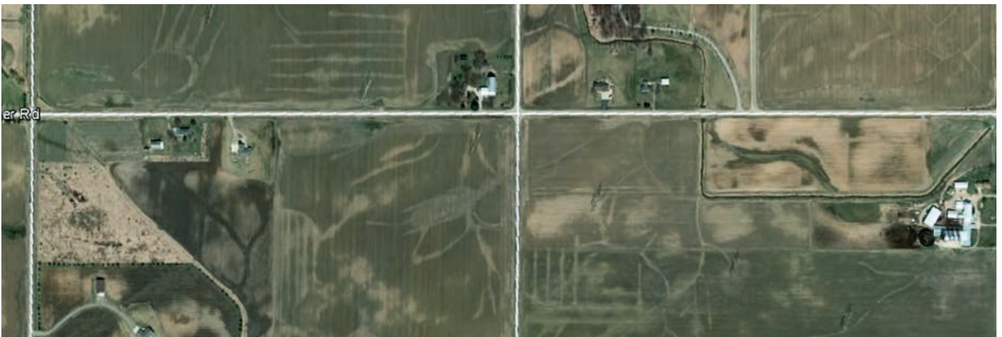
Figure 5. Satellite image revealing drainage systems
