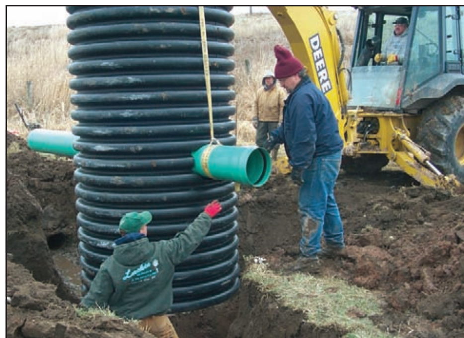
Figure 5. Tile monitoring equipment installation
