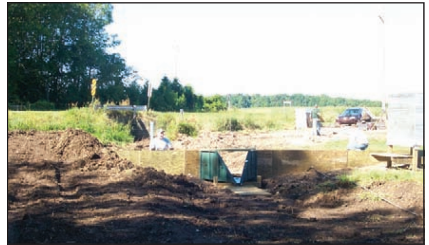
Figure 4. Upstream monitoring equipment install
