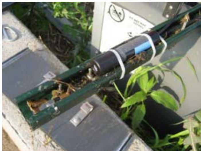
Figure 45: Decagon conductivity probe attachment at Farm B.
