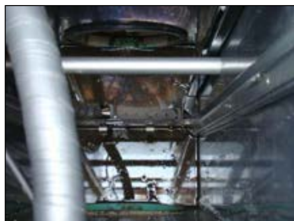
Figure 36: Sample line strainer attached to stoplog.
