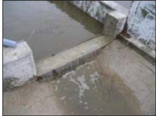
Figure 22: Final installation with flow.
