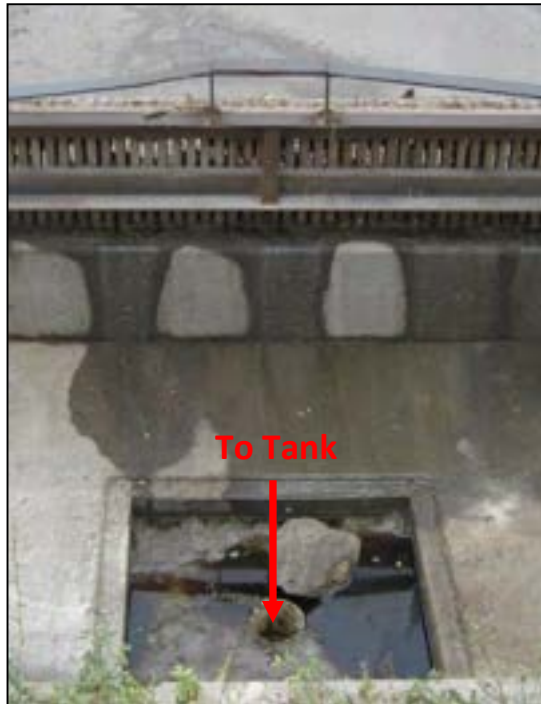
Figure 4: Leachate to collection tank.
