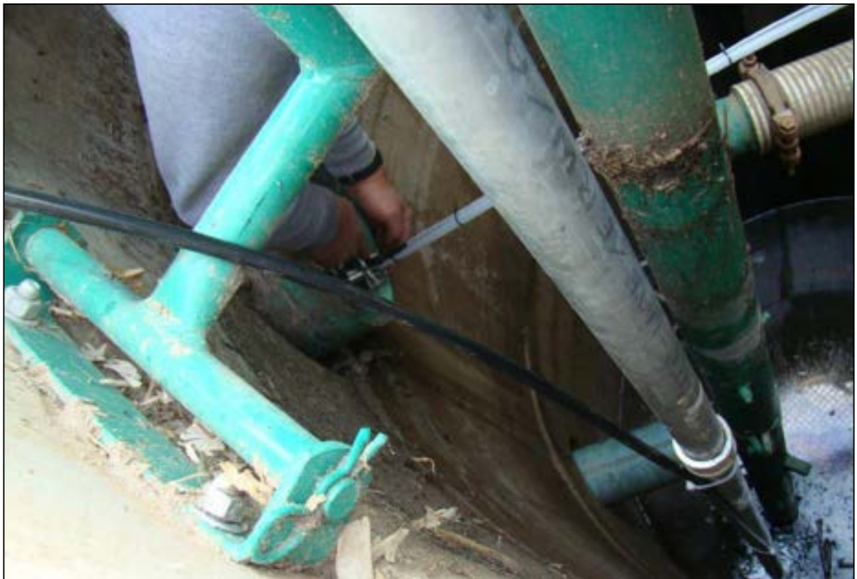
Figure 32: Sample and bubble lines installation and attachment on pipe.
