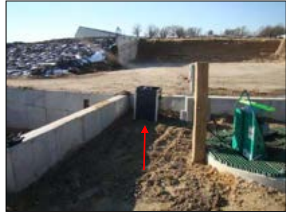
Figure 34: Installed Agri Drain.
