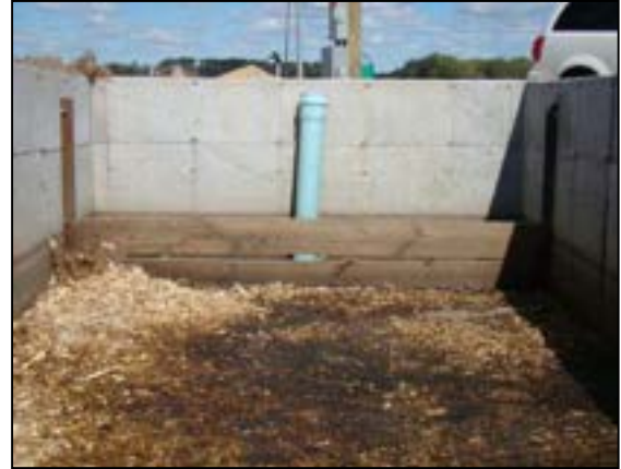
Figure 8: Wood pickets remove particles in the flotate trap.
