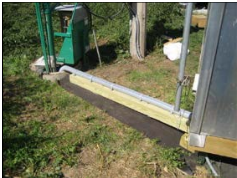
Figure 18: Final installation with protective ENT pipe.
