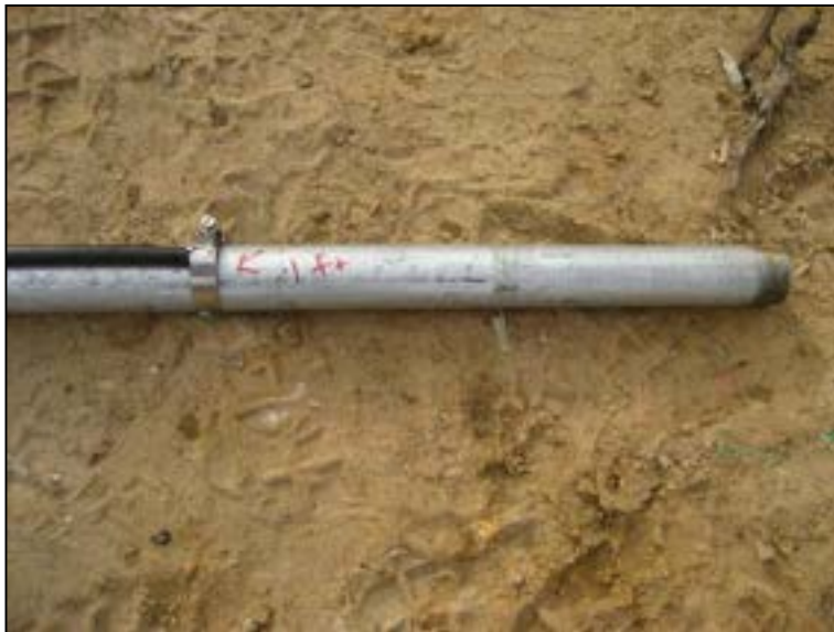
Figure 28: Bubble line placement on galvanized pipe.
